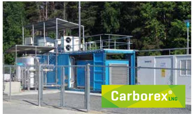
Carborex<sup>®</sup>MS plant in Jevnaker, Norway. With this DMT plant biogas is upgraded to pure methane. More references you will find when you visit our website [www.dmt-et.com/products](http://www.dmt-et.com/products). Here you will also find the animations "How does it work?"
